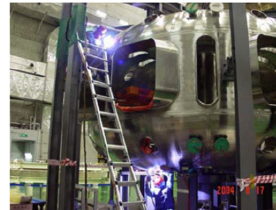
Fig. 12 Vacuum vessel under site welding
